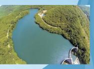
million m<sup>3</sup>. The reservoir is also equipped with a pumped-storage plant with a capacity of 1500 MW.
