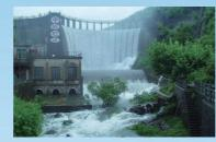
Pingqiao rock dam is located 2 km to the southeast of Tianmu lake. It was built in 1975, and is the largest masonry arch dam in Asia. The dam is 24 m high and 122 m long.
